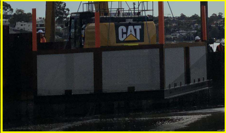
Ballasting with thin layer of sand with frame
